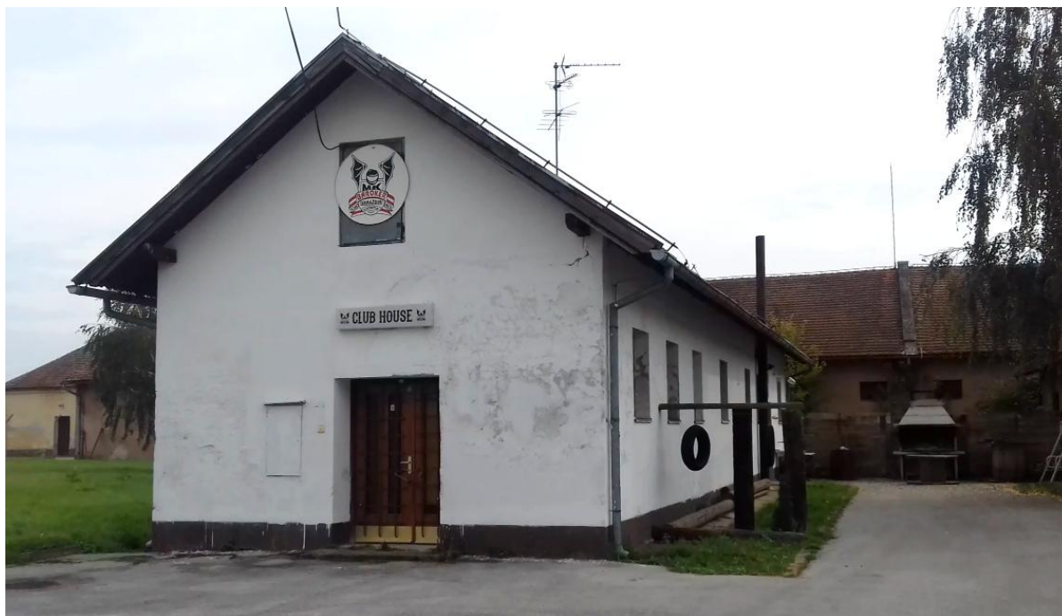
Picture 31 – building L
