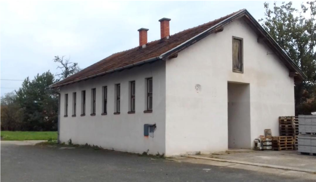
Picture 19 – building F
