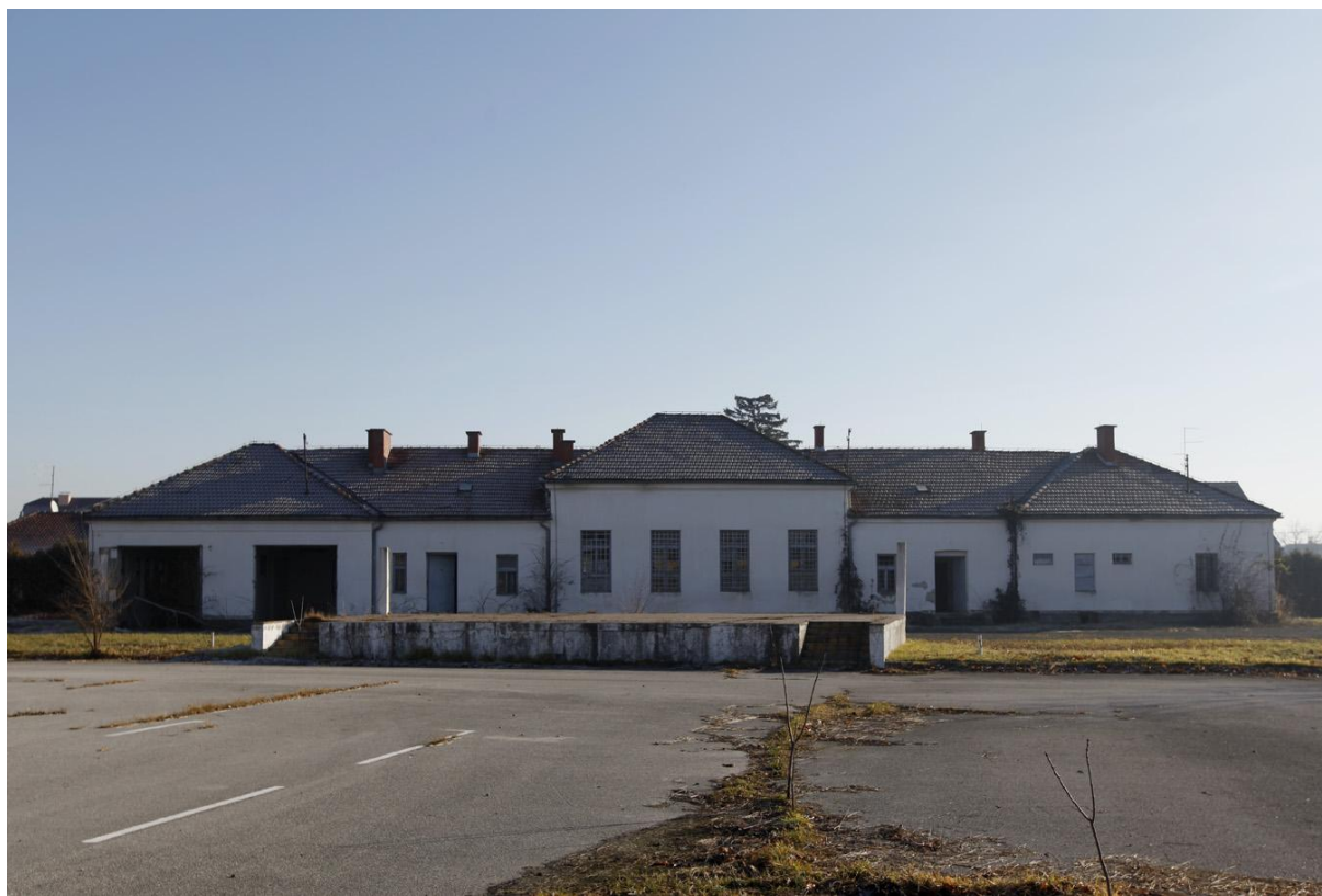
Picture 17 – building E
