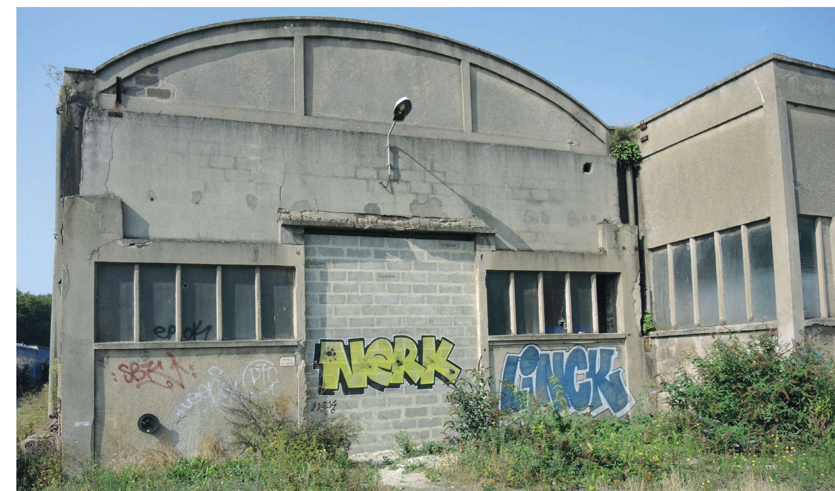
Priority: secure and preserve the building
