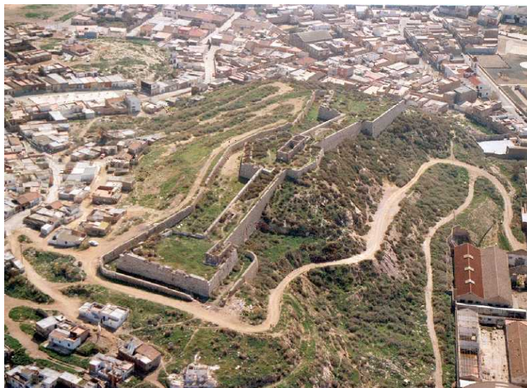
Figure 18. Open space area around the fortress
