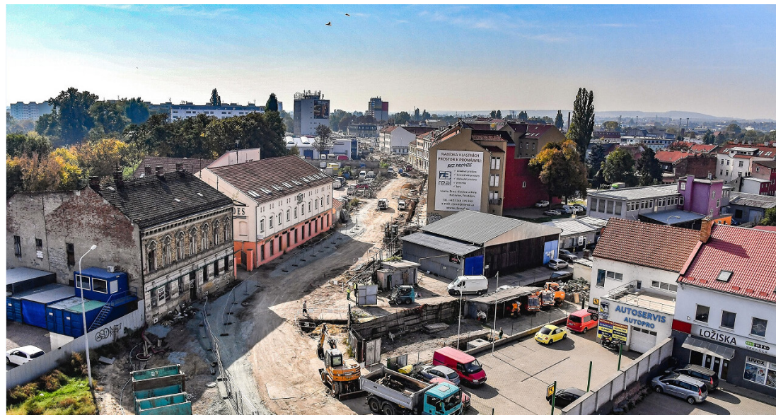
New tram line in Stavba-Dornych, Brno
