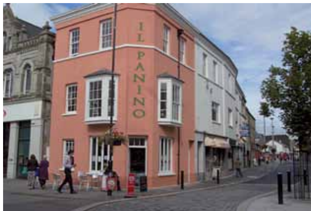
1-3 Market Street, Bridgend Townscape Heritage Initiative Scheme (BTHIS), Bridgend, UK.
