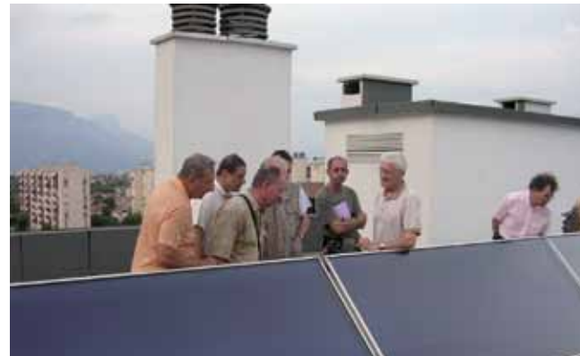
Chauffe-eau solaire (Echirolles, France)
