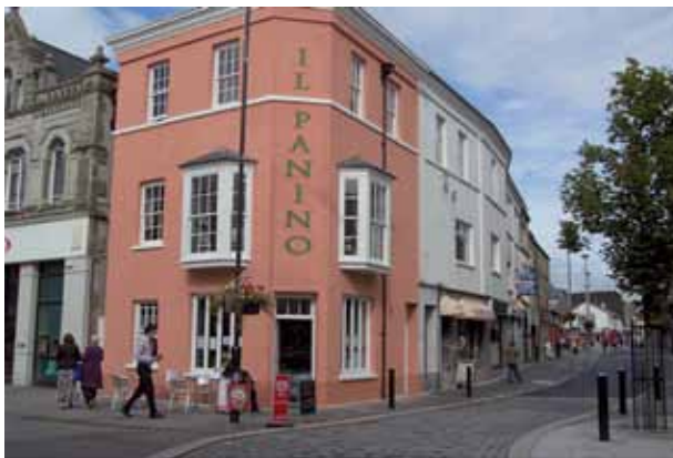
Market Street 1-3, Bridgend Townscape Heritage Initiative Scheme (BTHIS), Bridgend, UK.
