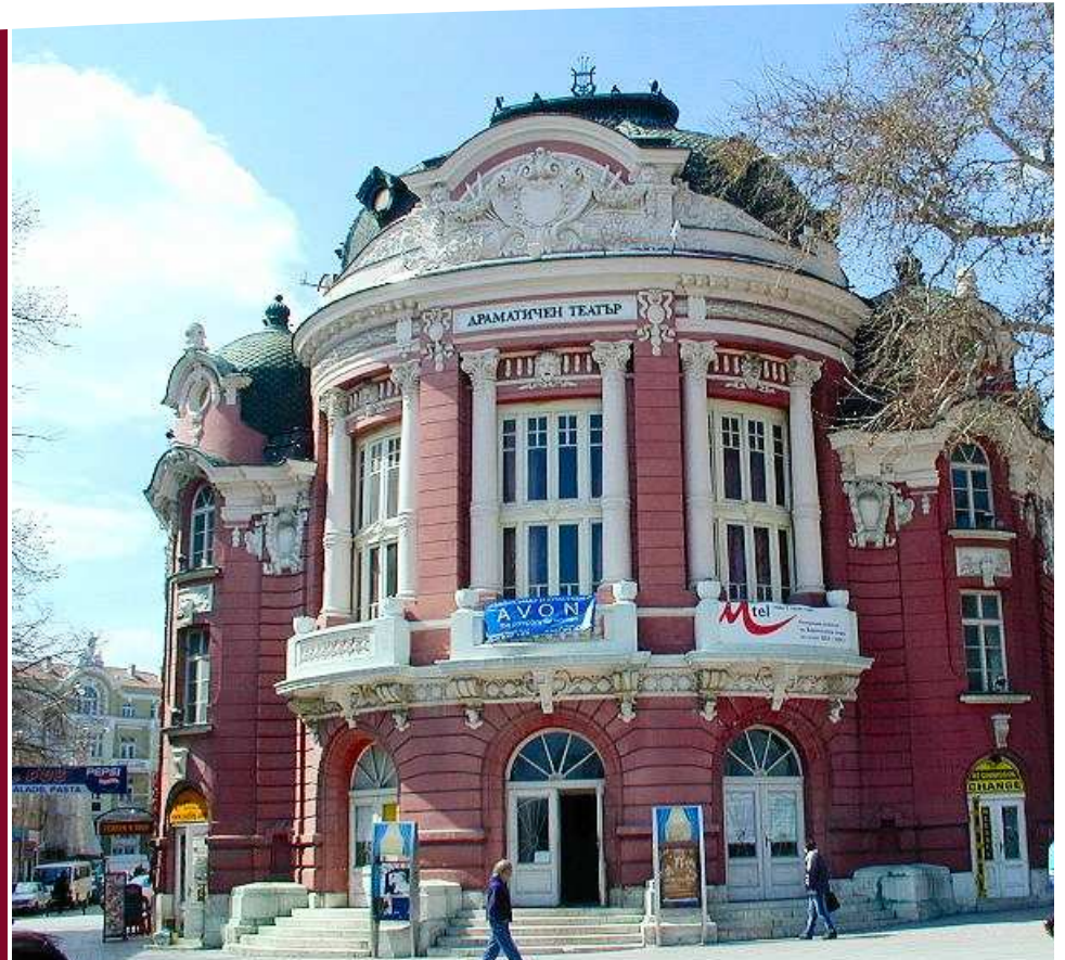
City of Varna. Photo Municipality of Varna
