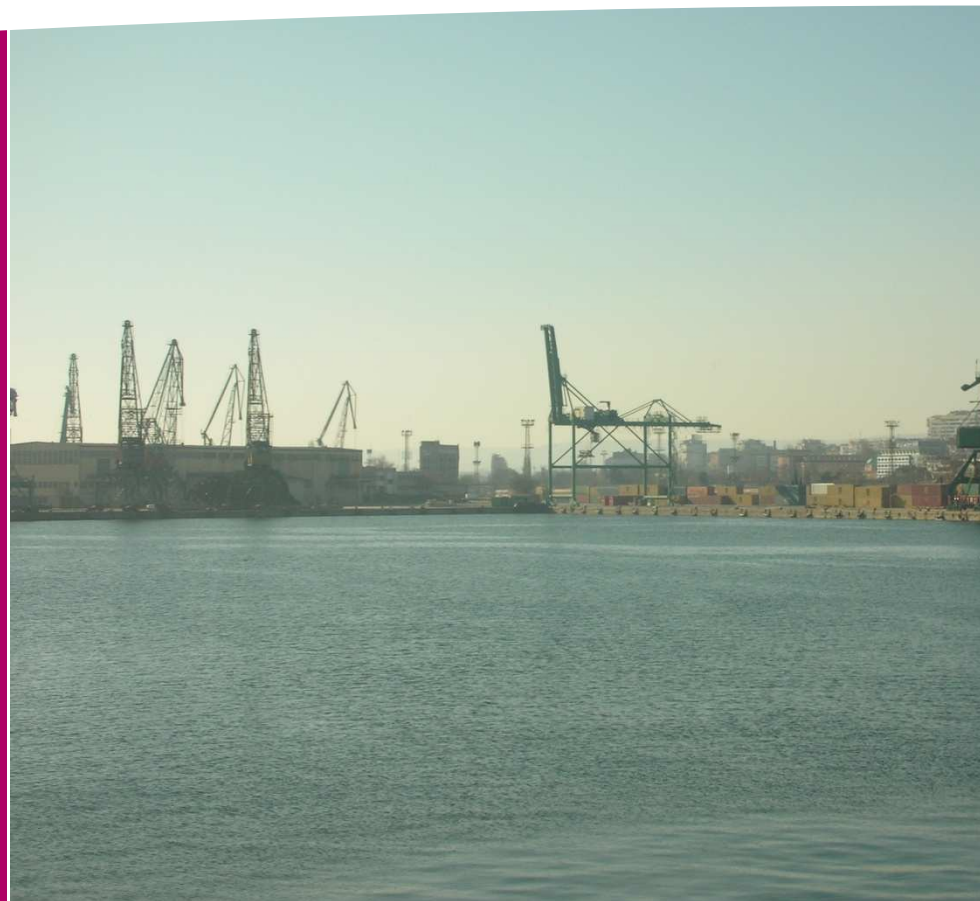
Varna port overview
