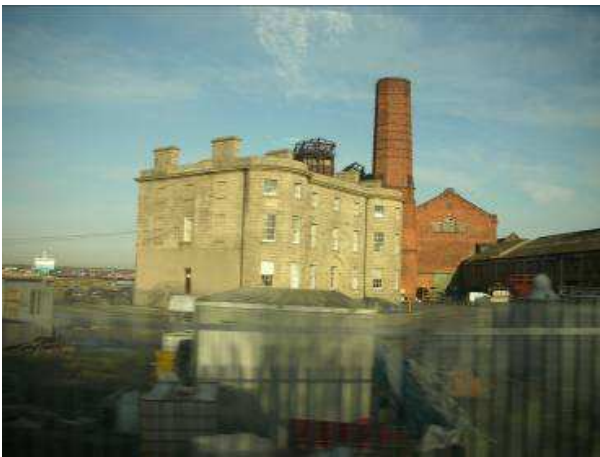
3. The former Poolbeg hotel. Photo P. Geoghegan
