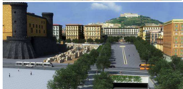
8. Infrastructures, connection port and city: the Piazza Municipio Station Project – Underground Line 1. Naples PPT
