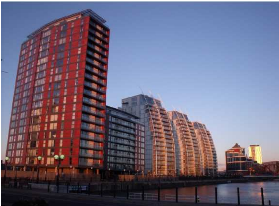
Figure 1: Huron Basin, Salford Quays
