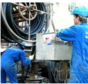
piping of the heat probes
