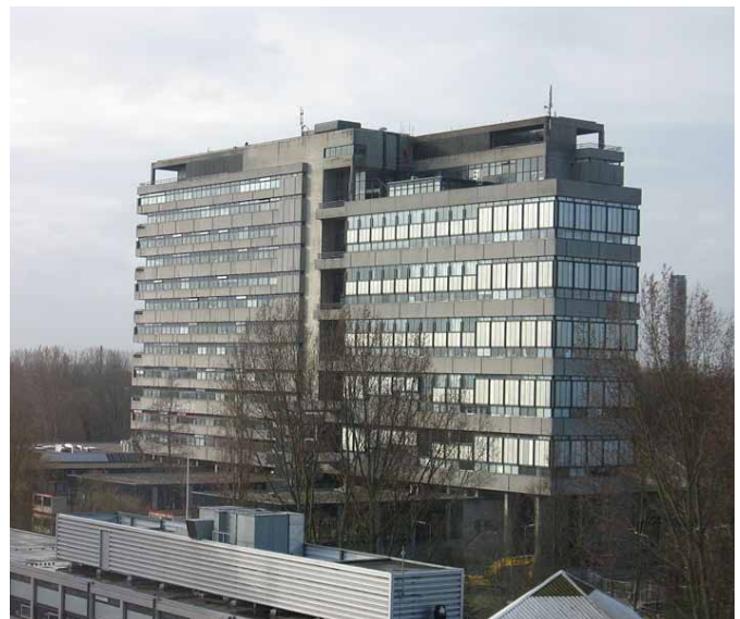
3. The former Faculty of Architecture (Van de Broek en Bakema)
