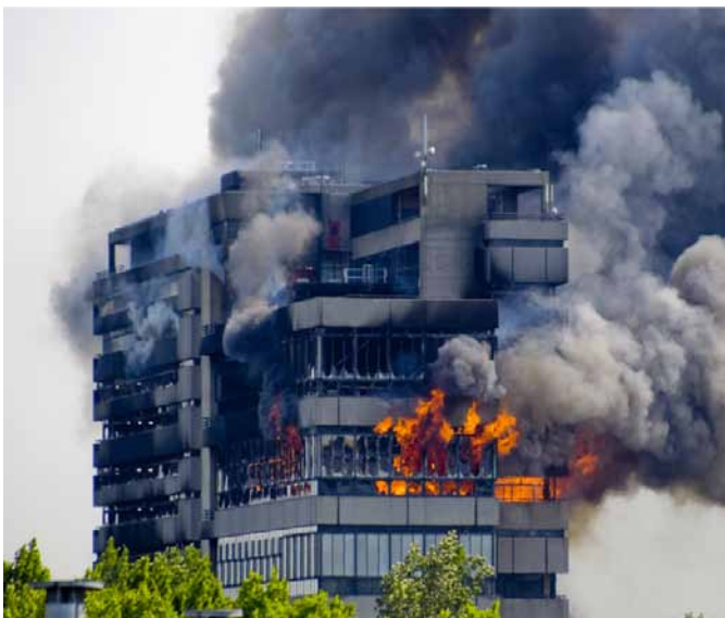
2. The Faculty of architecture on fire May 13 2008
