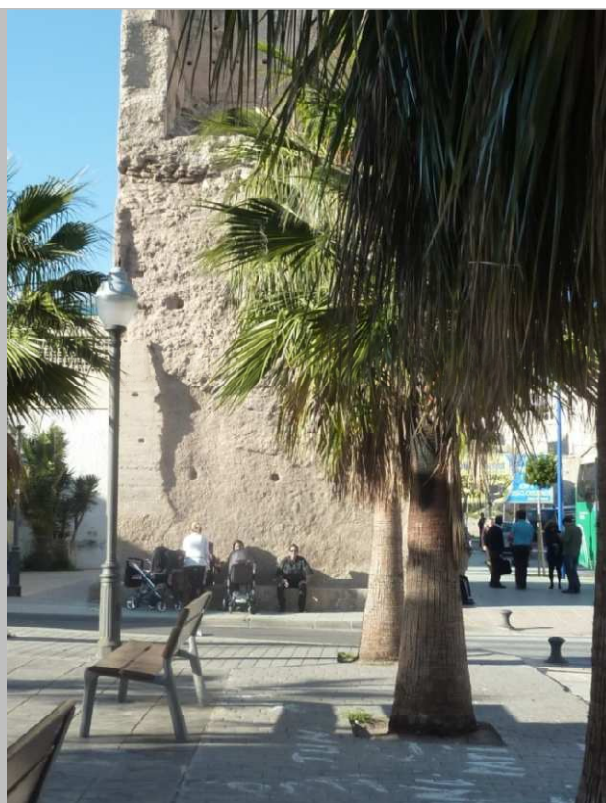
A vestige of the walls of 12th century
