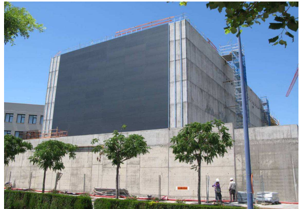
Ventilated façades of Jaume I University, Castellón
