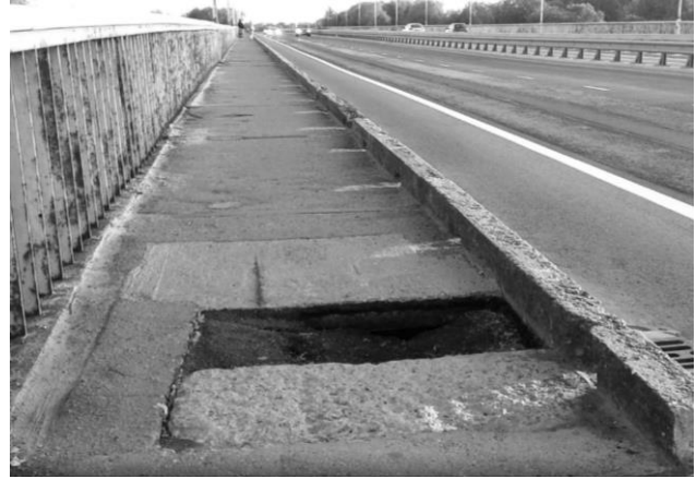
Illustration: a historical image of the completed bridge and its signs of amortization
