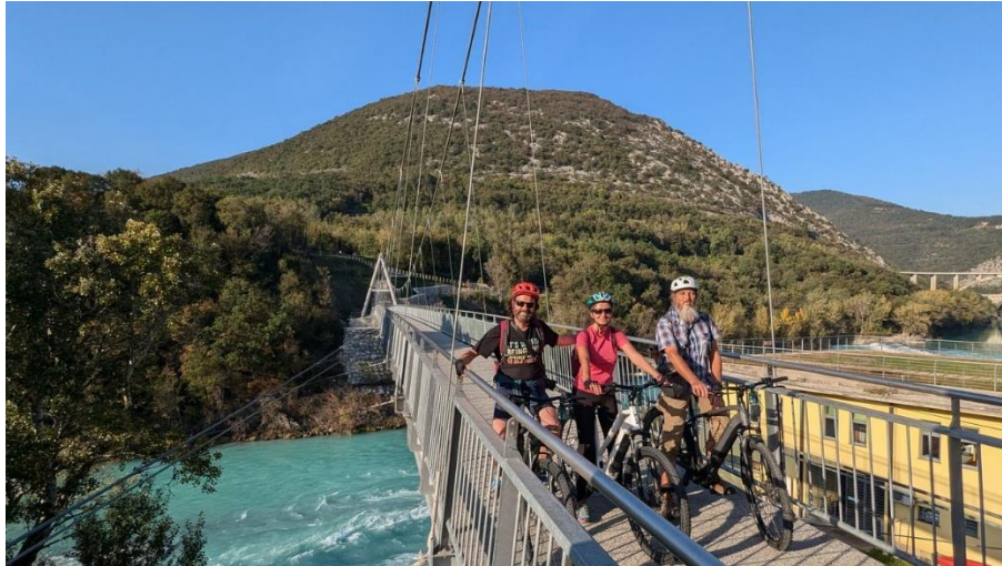
Cycling and pedestrian bridge over Soča/Isonzo river
