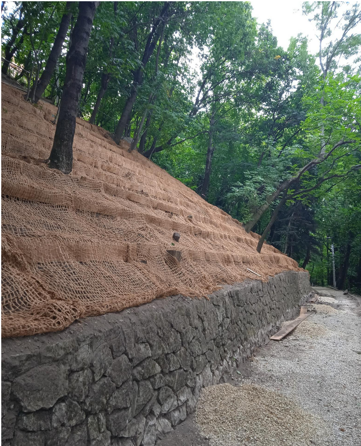
Figure 50 Coconut nets preventing soil erosion on steep rocky slopes (source: Practice Fiche)
