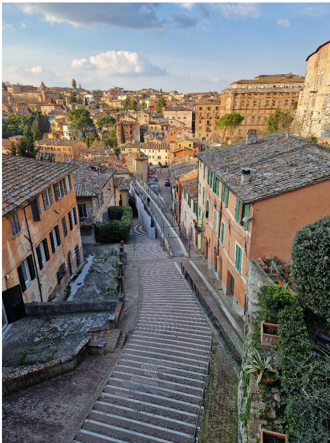
Photo: Perugia aqueduct.
