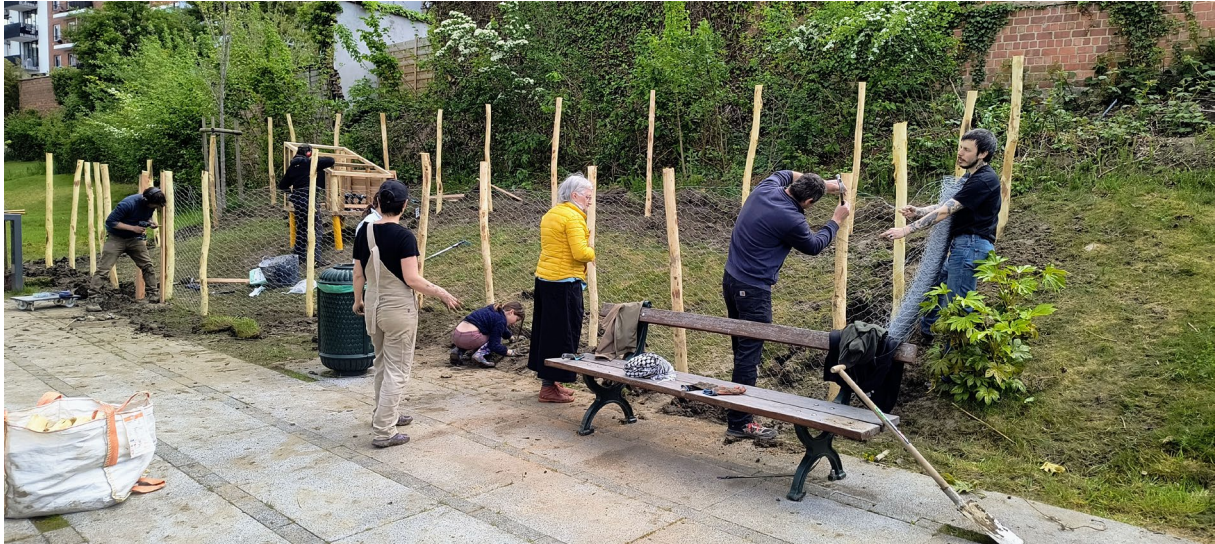
Photo taken during the participatory construction work, 18 April 2026 in Calico.
