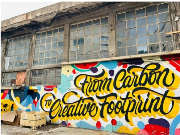
TUP factory in Dubrovnik visited during the Study Visit in November 2024
