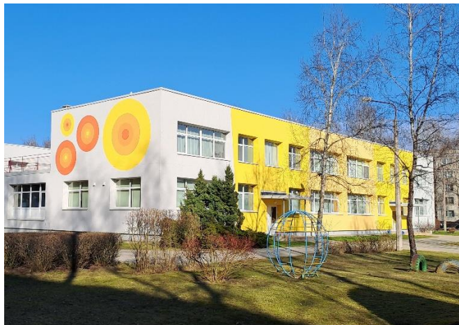
Marsa gatve 8 building
