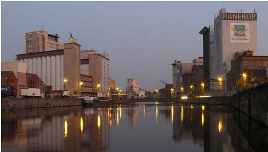
The industrial canal in Roeselare – May 2025
