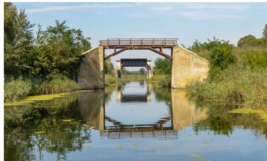
Figure 3: A bridge and old dam above the Great Bačka Canal (author: D. Siljanović Kozoderović).
