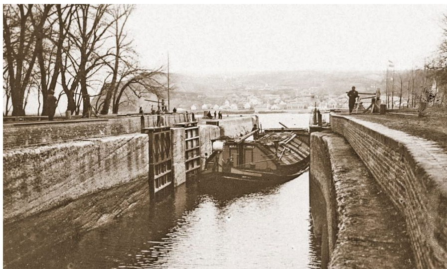
Figure 5: An old picture (from 1904) of the lock in Bezdan as the first example of underwater concreting in the whole world (source: www.ravnoplov.rs / Milan Stepanović).
