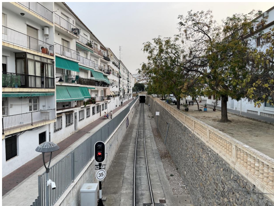
Physical rupture separating neighbourhoods of Altea. Photo by Levente Polyák
