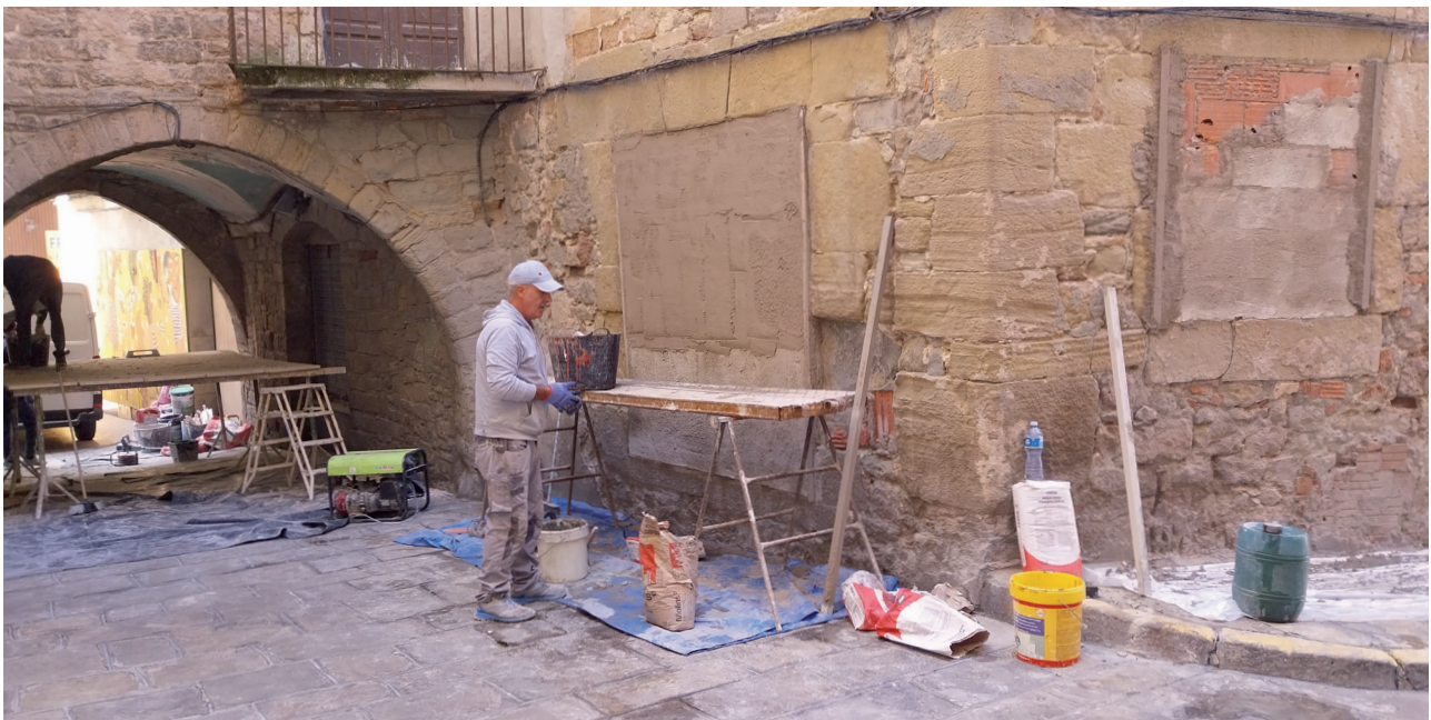
Figure 13: Public space renovation works in Manresa. Source: Municipality of Manresa
